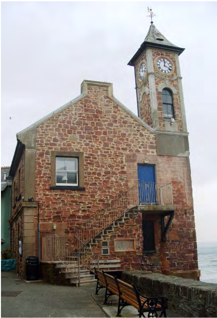
Above: Kingsand Institute and clock tower, Cornwall. Constructed from Kingsand rhyolite and sandstone with Devon Limestone dressings
