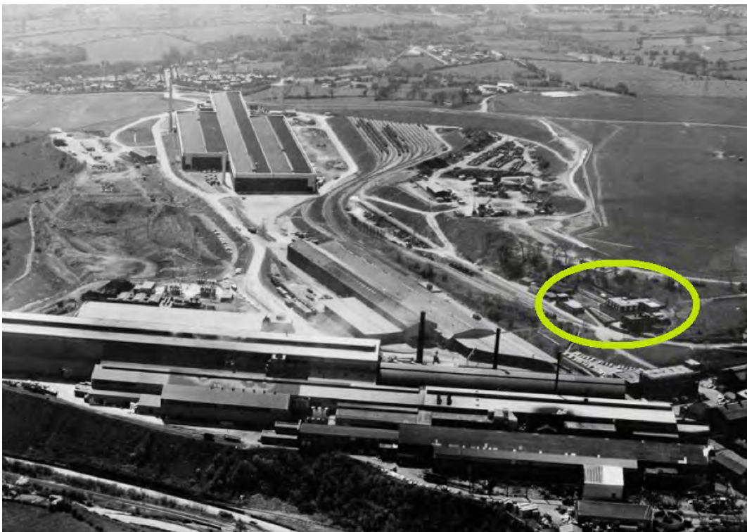
Brymbo Steelworks in 1990. A vast complex of buildings with the oldest structures dating from the late 18 th Century. The Fossil Forest was discovered beneath the former office block (marked). Photo courtesy of Brymbo Developments Ltd.
