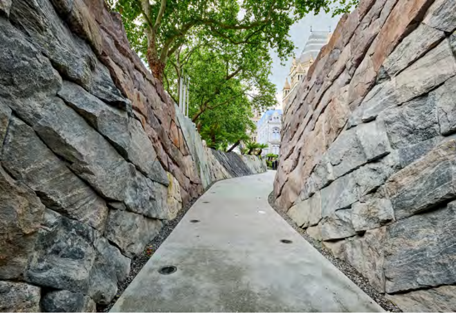
The Transport for London tunnel entrance opens into a canyon clad in our most ancient Precambrian rocks from Scotland.
